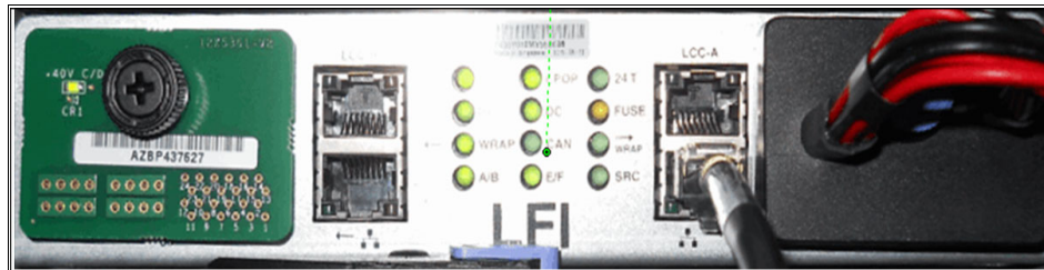
Figure 1-46 Library frame interconnect
