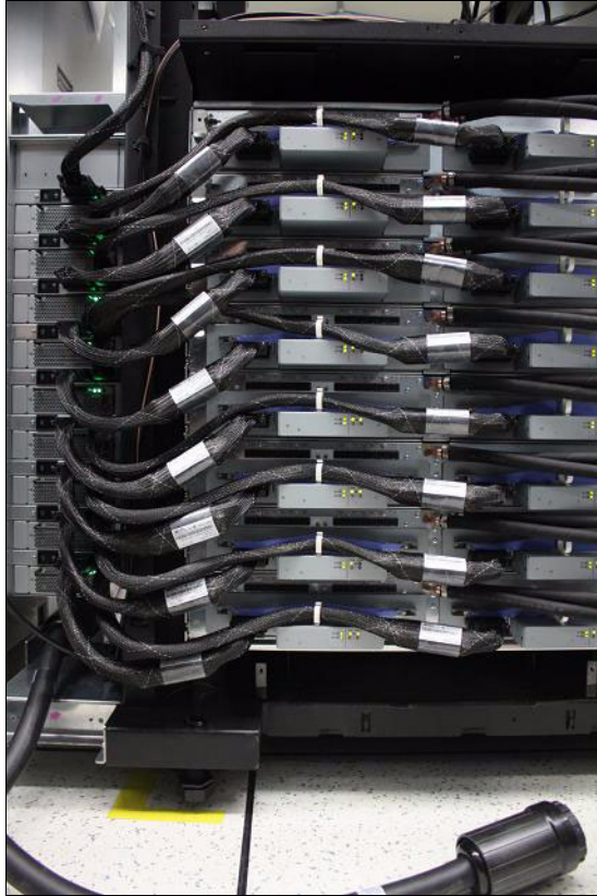
Figure 1-26 Completed BPE to DCA cabling
