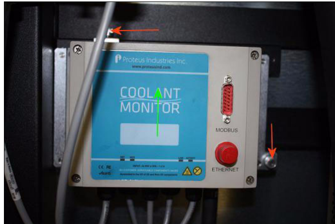
Figure 4-39 Coolant monitor removal 4
